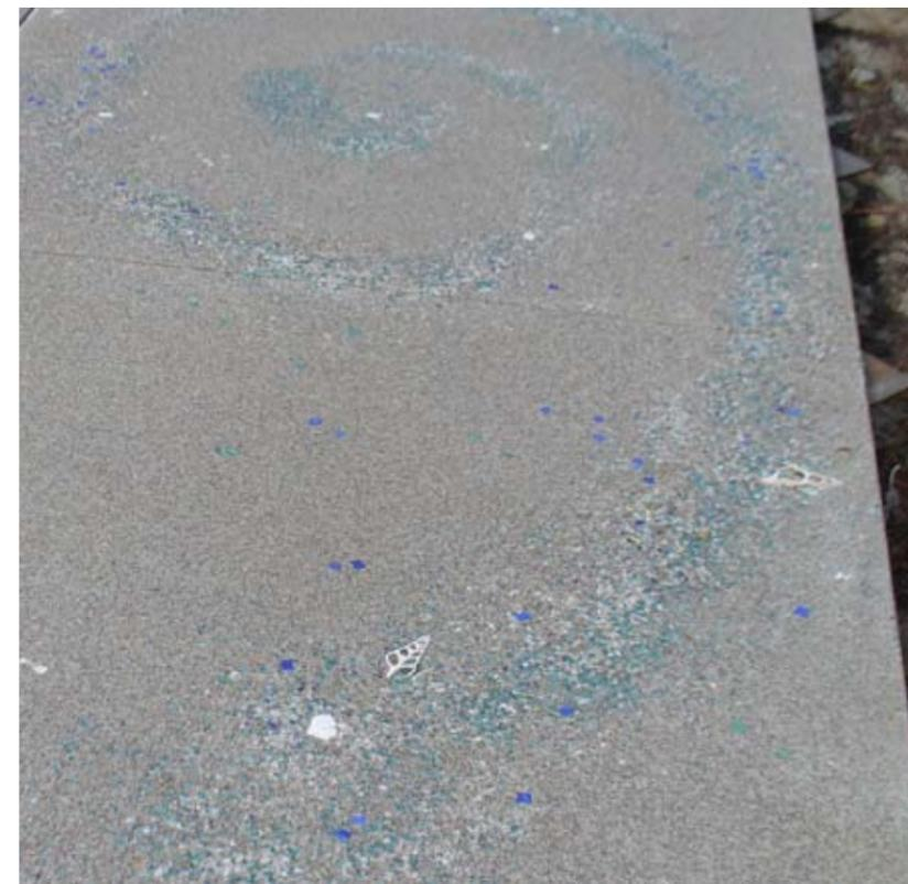
Example of decorative aggregate inlay using tumbled glass and shells in concrete. This can spotlight graphic motifs described further in the Signage section.
