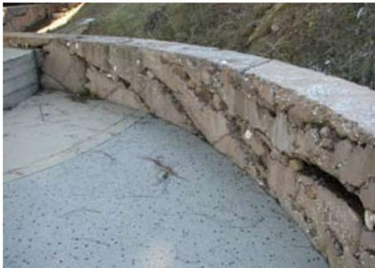
Example of a concrete seatwall that has been poured for a unique appearance.
